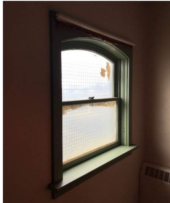
Plate 81: Original window and moulded wood surround on the third floor
