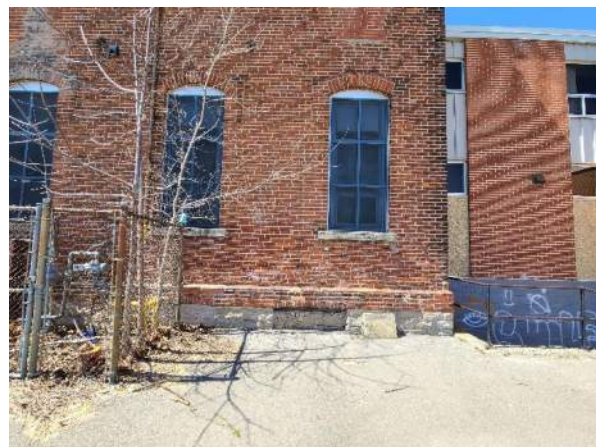
Plate 56: Segmentally arched windows on the rear elevation of the original school
