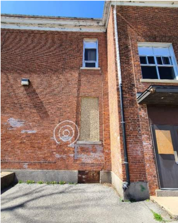
Plate 59: Photo of concrete foundations, red brick exterior, and rectangular windows on the 1921/1924 addition
