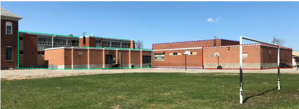
Plate 48: Northwest view of the east elevation of the College Street Public School showing the 1959 addition (outlined in green), 1967 addition (outlined in light blue), 1969 addition (outlined in purple), and 1972 addition (outlined in red)
