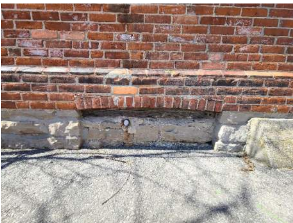
Plate 55: Stone foundations and red brick exterior of the original school
