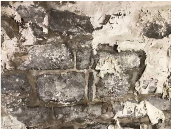
Plate 83: Detail of stone foundations in the 1885/1887 section of the basement
