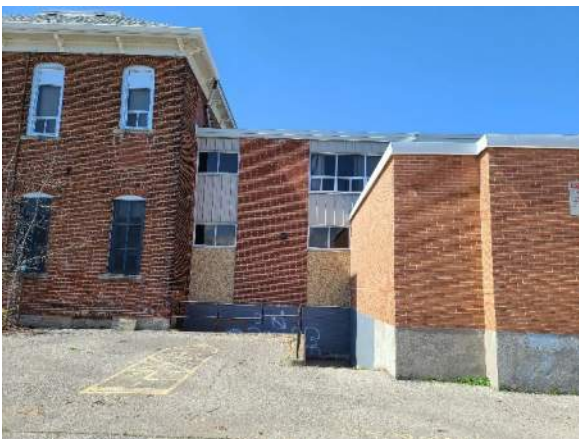
Plate 49: East elevation of the 1959 and 1969 additions showing the below grade access to the basement
