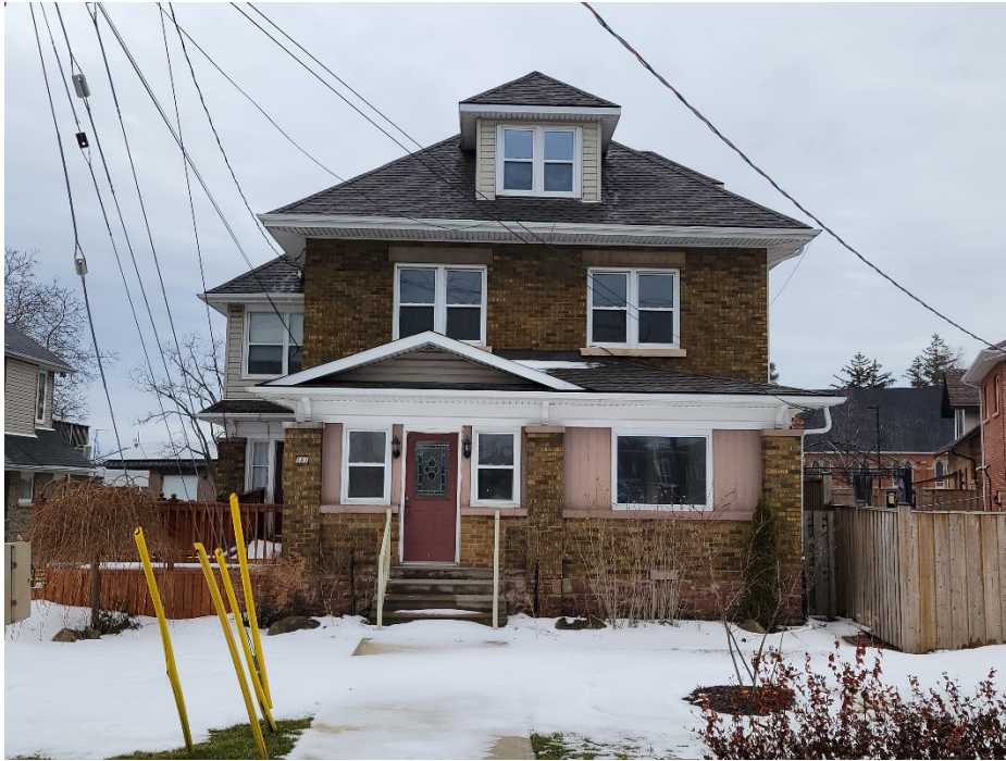
Photo 1: Subject Lands - Main Building
