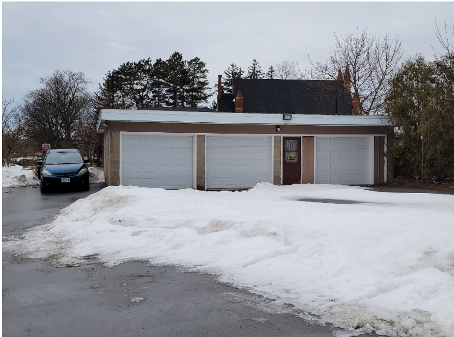
Photo 2: Subject Lands – Garage at Rear
