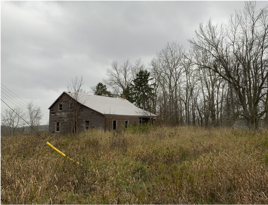
Photo 2: Looking south, abandoned residence located North of the Creek, fronting on Range Road 2
