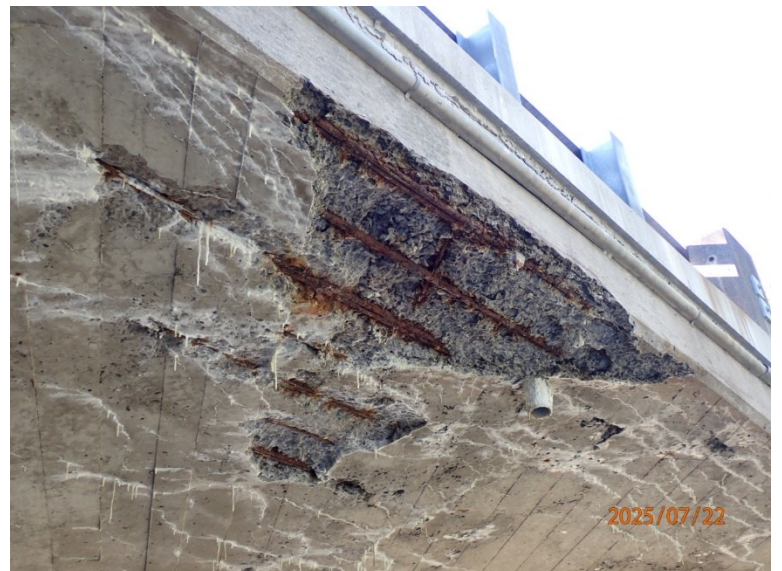
Figure 94 Photos of a culvert in 'poor' condition: Roy Bridge
