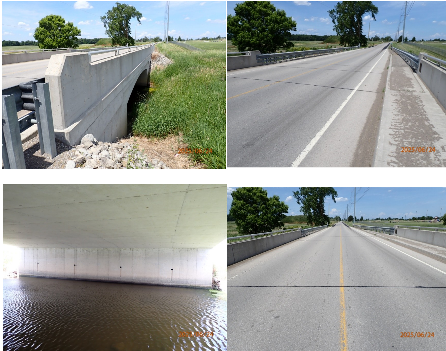
Figure 92 Photos of a bridge in a 'very good' condition: South Grimsby Road
